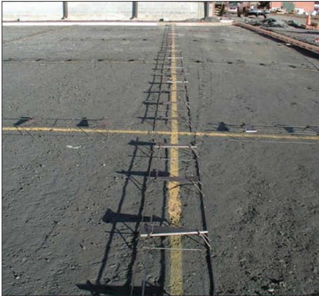
One of the earliest uses of tapered plate dowels was this pavement section at the Atlanta Bonded Warehouse distribution center in Kennesaw, Ga. After four years of constant truck traffic there is no damage at the contraction joints even though the slab is only 6 inches thick
