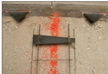
Fig. 8—Tapered plate dowel spacing example for a 4000-pound standard lift truck on a 6-inch-thick slab.
